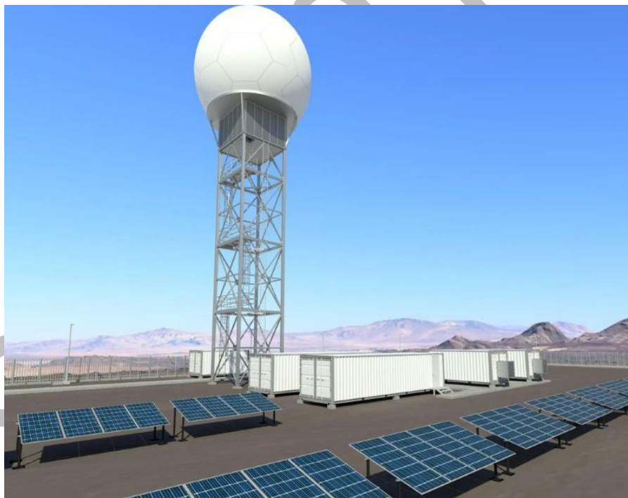
Figure 6: Solar powered radar system
